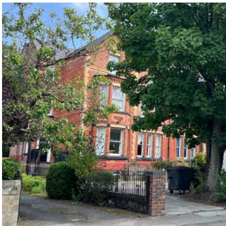
Residential properties along Park Road
