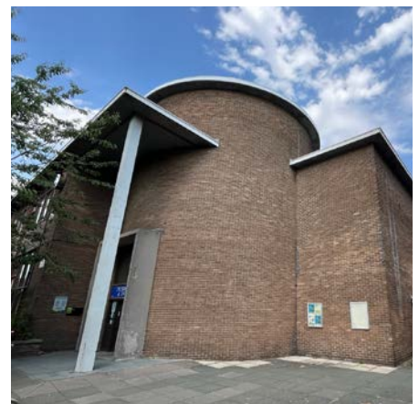
Existing library and civic centre buildings to be demolished
